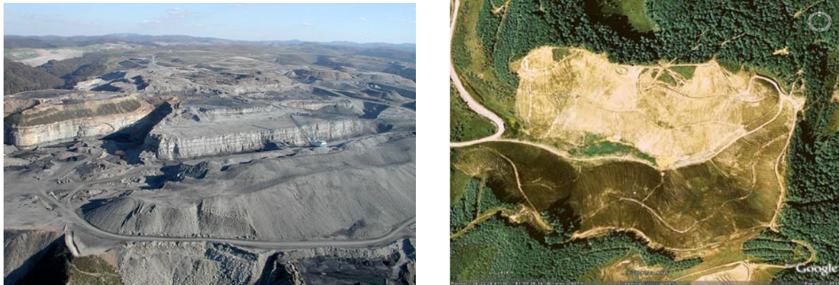
(A) A view of a mountain top operation rock face. (B) An aerial view of a completed mining
